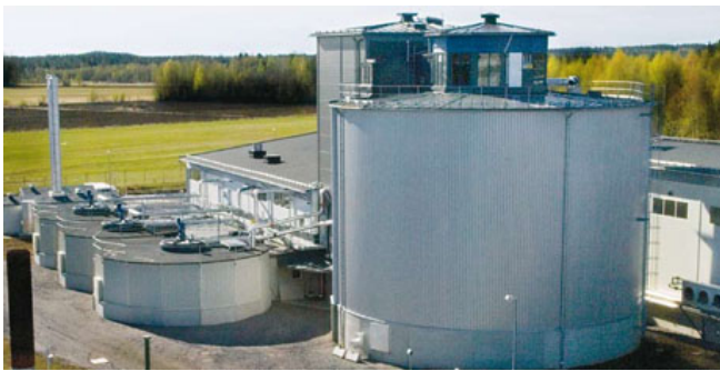
Figure 8C4: The biogas plant at Ön's waste water treatment plant, supplying the plant and UMEVA's offices with electricity and heating.
