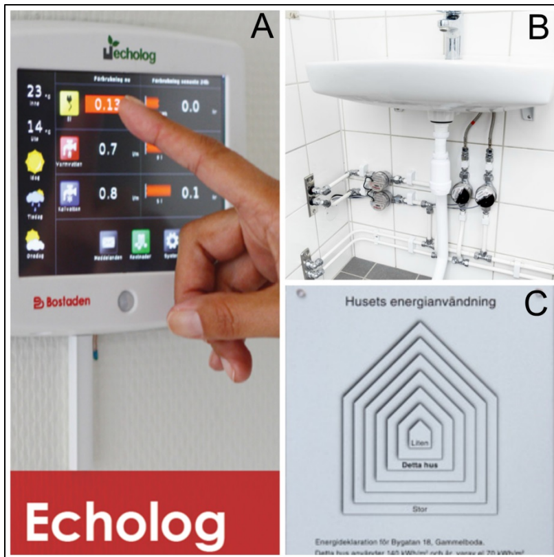
Figure 8B1: (A) The terminal “Echolog” in all Bostaden’s new apartments shows the consumption of electricity and hot and cold water in real time. The purpose is to help reduce consumption through increased awareness. (B) “Intelligent” equipment as used in the pilot study. (C) Energy performance graph from low to high performance (in the middle) according to which properties are classified. (Photo source: (A) Bostaden; (B) FM Mattson)
